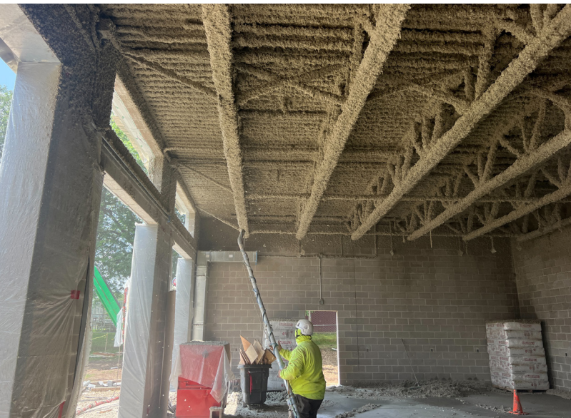
FIREPROOFING APPLIED TO JOISTS
