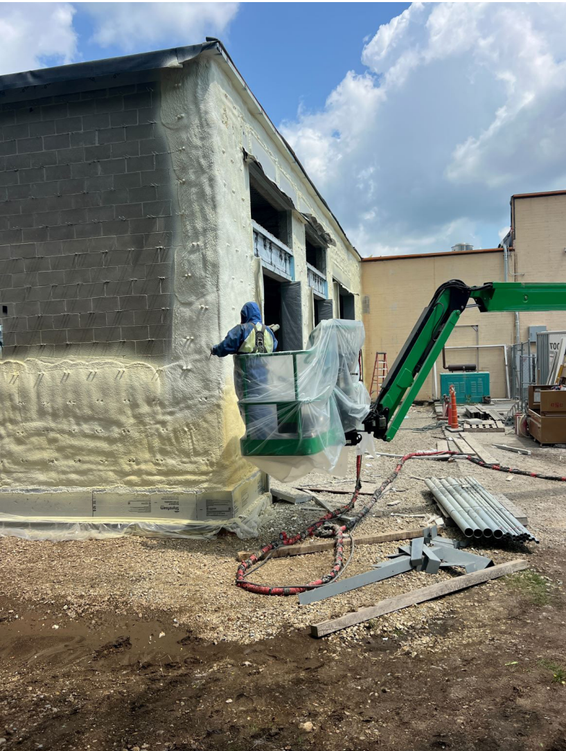
SPRAY FOAM BEING APPLIED TO CMU
